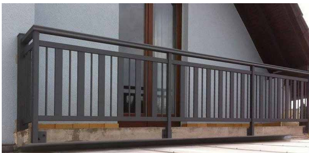
Pose sur dalle + poteaux d'angle 100x100 mm
