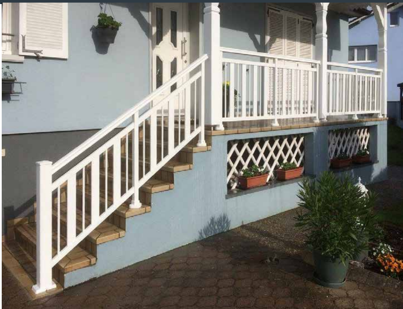
Pose sur dalle + poteaux d'angle 100x100 mm
