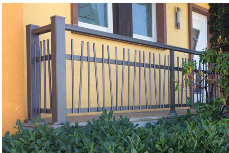
Pose sur dalle + poteaux d'angle 100x100 mm
